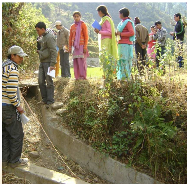
Audit committee checking the canal construction
